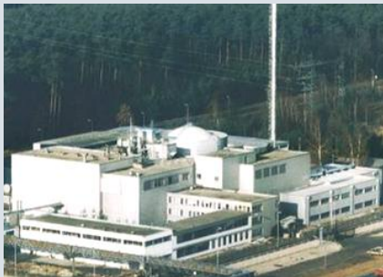
Prototype for advanced fast reactor cooled with liquid sodium
