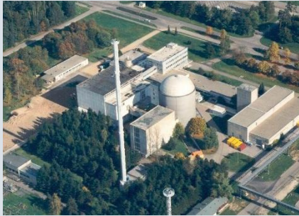
Prototype pressurized heavy-water reactor (PHWR)
