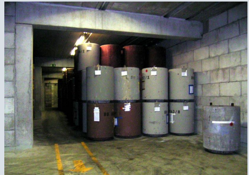
storage chamber with concrete-shielded casks
