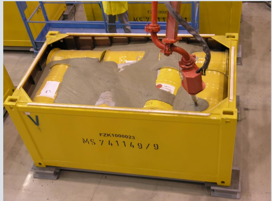
cementing of containers
